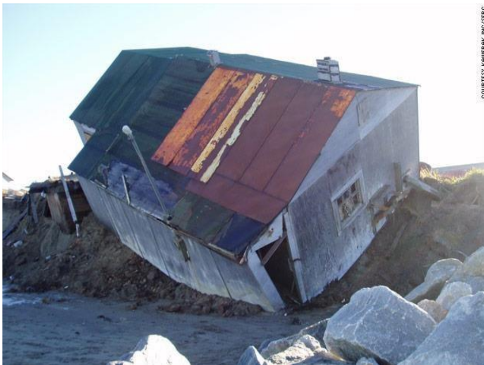
Figure 34: Coastal Erosion in the Native Village of Shishmarof, Source: John Sutter, CNN
